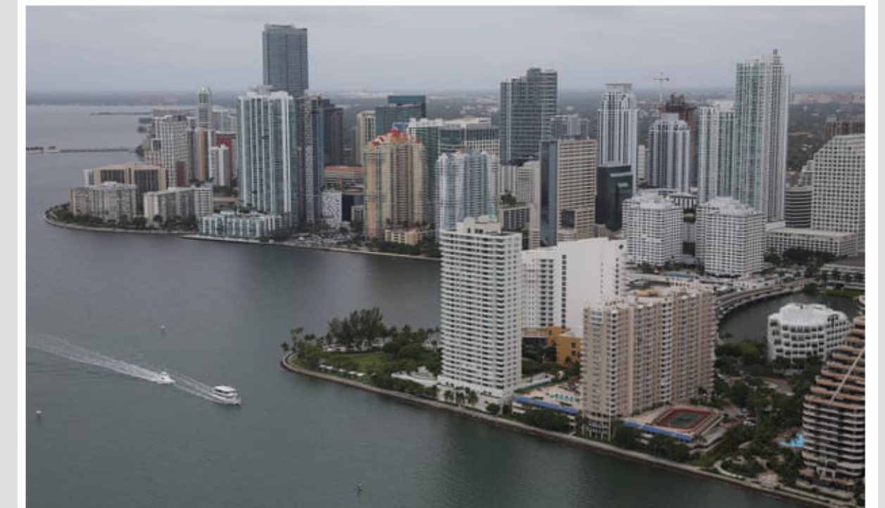
▲ Waterfront condo buildings are seen June 3, 2014 in Miami, Florida. Photograph: Joe Raedle/Getty Images
