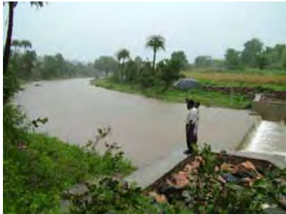
(a) Anicut under construction June 2004 (pre-monsoon) (m)
