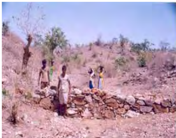
(a) LSCD under construction June 2004 (pre-monsoon)
